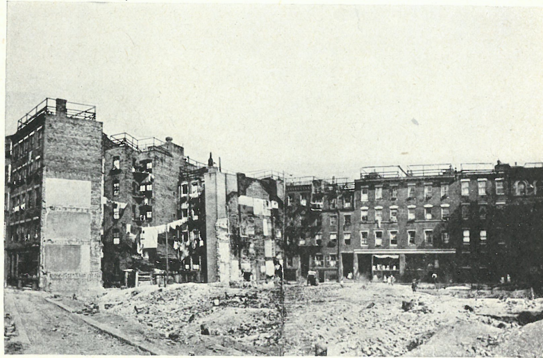
FIG. 41.—THE NORTH END. PHOTOGRAPH SHOWING AREA WHERE BUILDINGS HAVE BEEN TORN DOWN IN MORTON STREET DISTRICT TO MAKE ROOM FOR PLAYGROUND DEVELOPMENT.
