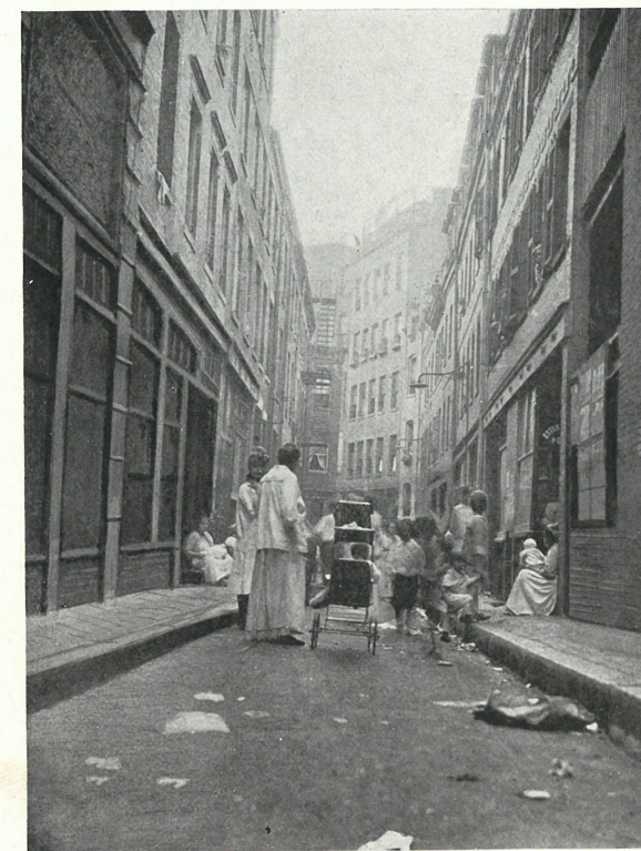
FIG. 36.—VIEW OF MORTON STREET, LOOKING WEST FROM SALEM STREET; 11 TO 14 FEET BETWEEN WALLS. 1915.
